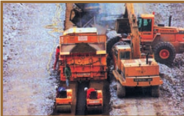
The placing machine in operation
