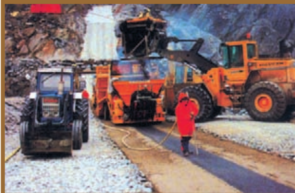
Cleaning the previous layer
